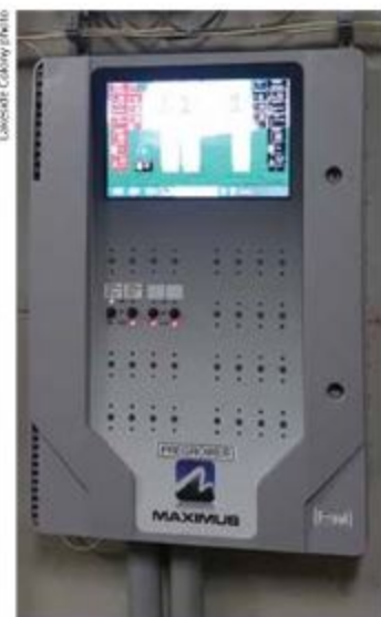
The Lakeside Colony near Lethbridge, Alta., installed the Maximus controller system last year, and staff already see it as a game changer for their hog business.
